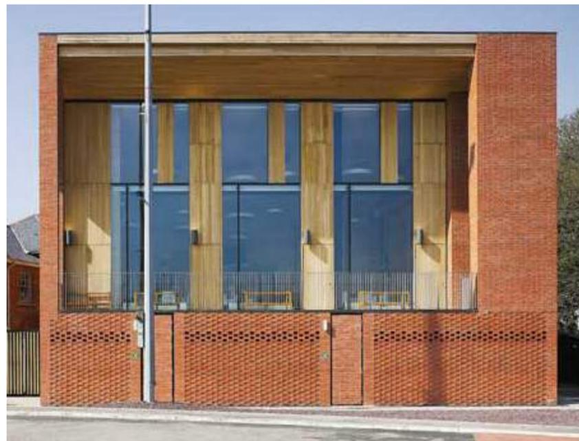
Window frames are to be recessed behind the brick or timber reveals where possible - to assist the thermal performance and provide a clean finish. Windows will have the same colour of aluminium outer facing as the curtain walling system.
