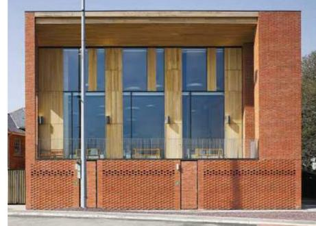
Window frames are to be recessed behind the brick or timber reveals where possible - to assist the thermal performance and provide a clean finish. Windows will have the same colour of aluminium outer facing as the curtain walling system.
